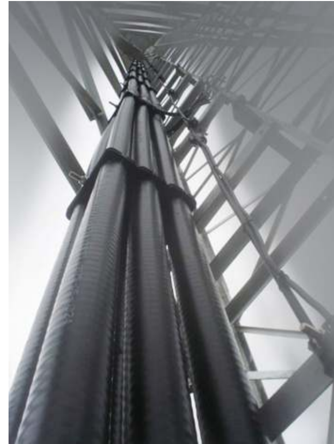
Corrugated Coax Cables
