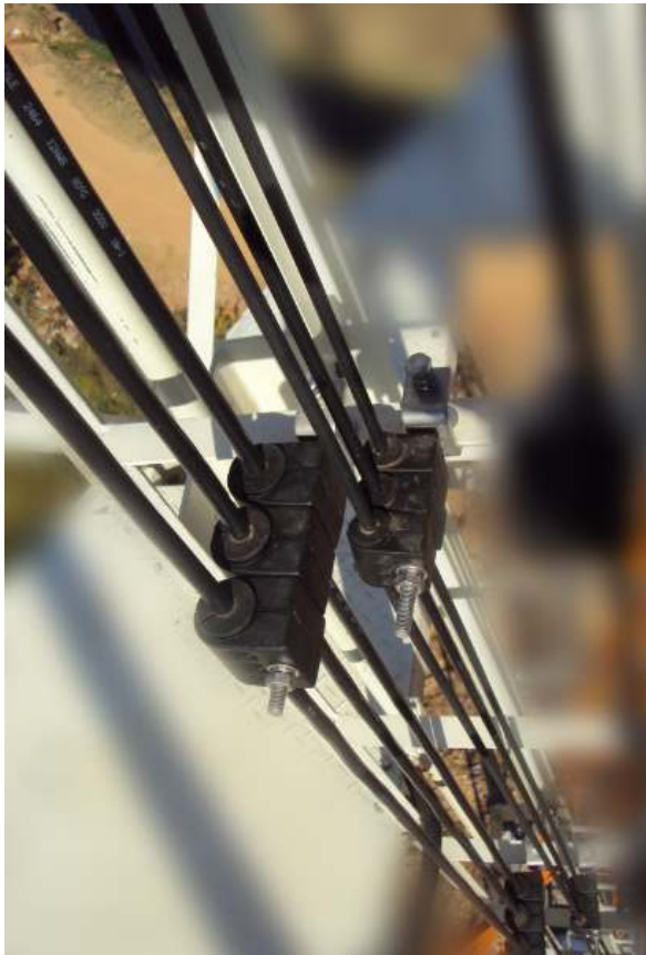
Optical and Power Cables (Conventional)
